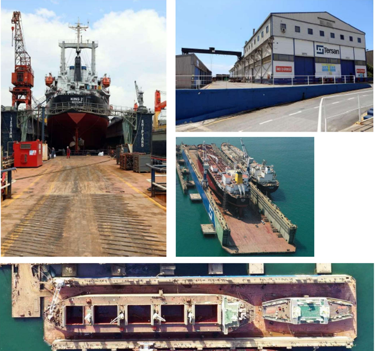
FIGURE 2. GENERAL OVERVIEW OF EXISTING FACILITIES OF TERSAN
